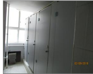
Photo of the sanitary facilities Toilet.JPG
