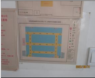
Photo of fire safety equipment Fire emergency evacuation map.JPG
